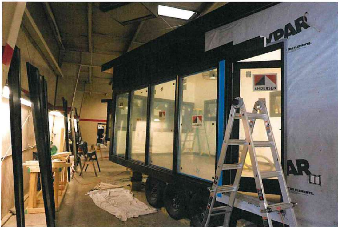
TimberHut says it utilizes higher-end building materials, like Anderson windows, to make the units as maintenance-free as possible.
