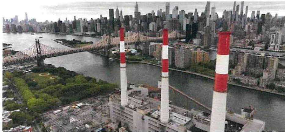
Astoria's Ravenswood Generating Station. LOKMAN VURAL ELIBOL/ANADOLU AGENCY VIA GETTY IMAGES
